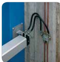
Connection to the 6-way oil pipe block
