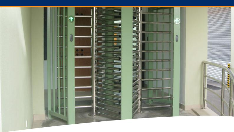
If you want to be 100% sure of reliable site access security then the full-height Electro Sesame Twin full height turnstile is the best choice. This device provides complete access control being a physical barrier, subject to the required level of security it can be supplied with either a single or double cage.
